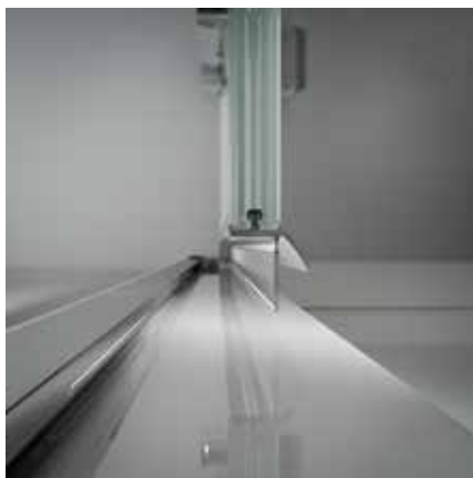
Water repellent profile in groove without clamping surface
