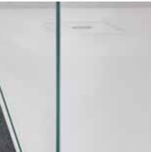
○ Glued glass-glass connection (not mitred)
